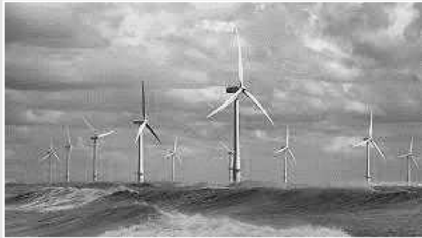
Figure 1: Wind installations with collinear turbines.
