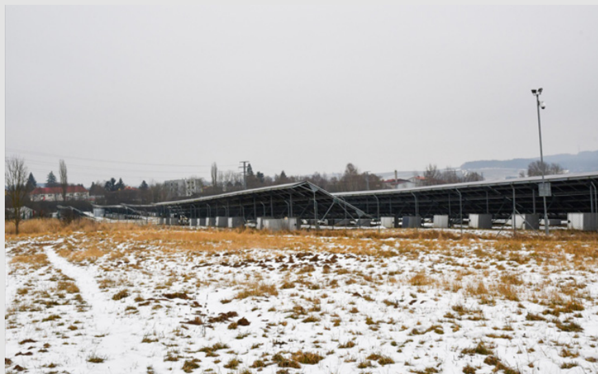
Figure 1: Ground photovoltaic power plant in Stříbro-photography by Tomáš Hájek -2026-postproduction by Petr Zajíček. Start of operation in 2009, installed output 13.6 MW. The solar park with its total mass makes a significant impression, but none of the strategies for contextualization of a solar park in a landscape is used. The photographed part of the solar park is situated in an industrial zone of the historical town of Stříbro, where the concealing strategy would probably be suitable. In general, the town of Stříbro has a unique genius locus and is situated in an undulating landscape, which allows for interesting lookouts to be created.
