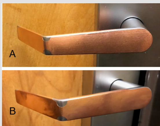
Figure 1: Dorm room handle. A is immediately after copper installation. B is 1 month later.
